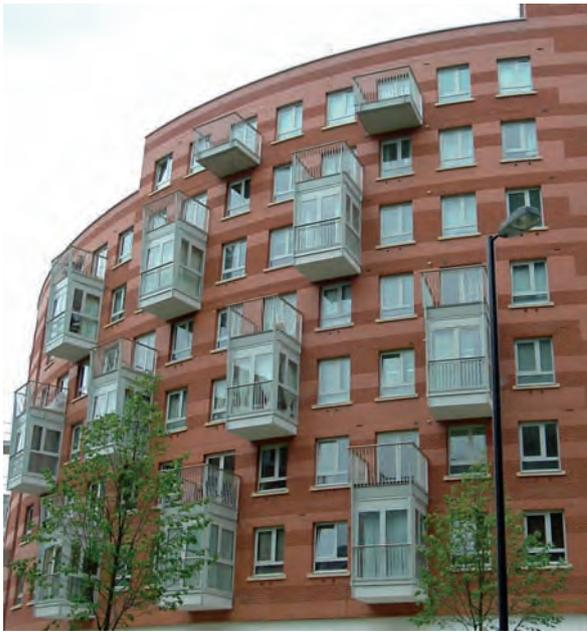
Figure 13: This North London development (architects CZWG) has staggered balconies to minimise obstruction to living rooms. Where a balcony is above a living room the obstructed area has been modified to form an unobstructed bay window.
