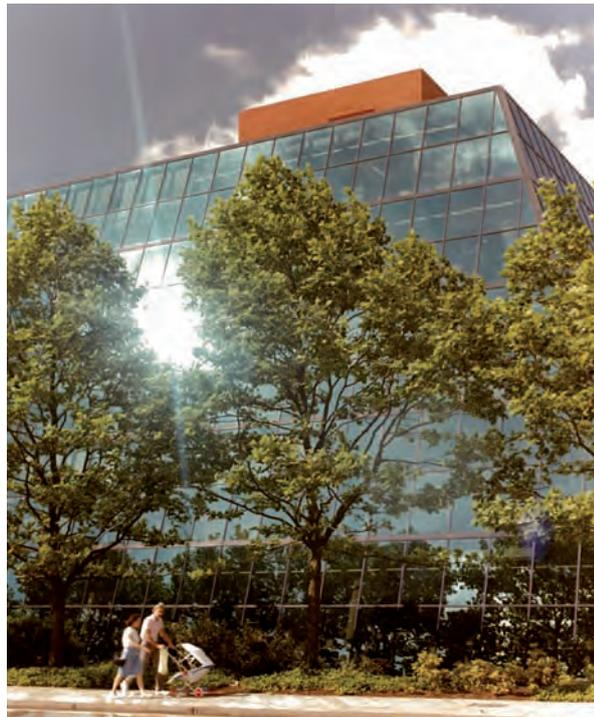
Figure 39: Solar dazzle reflected from a glazed façade
