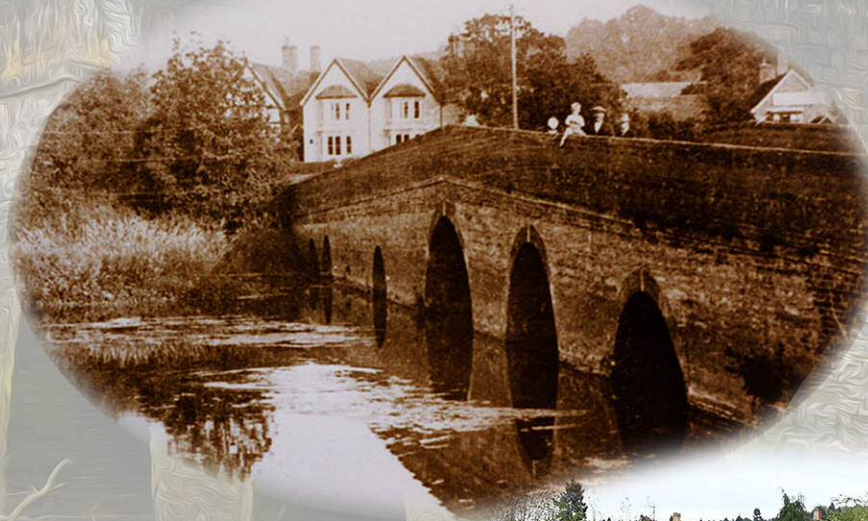
Oversley Bridge circa 1910. Note narrow tunnels to left of central arch.
