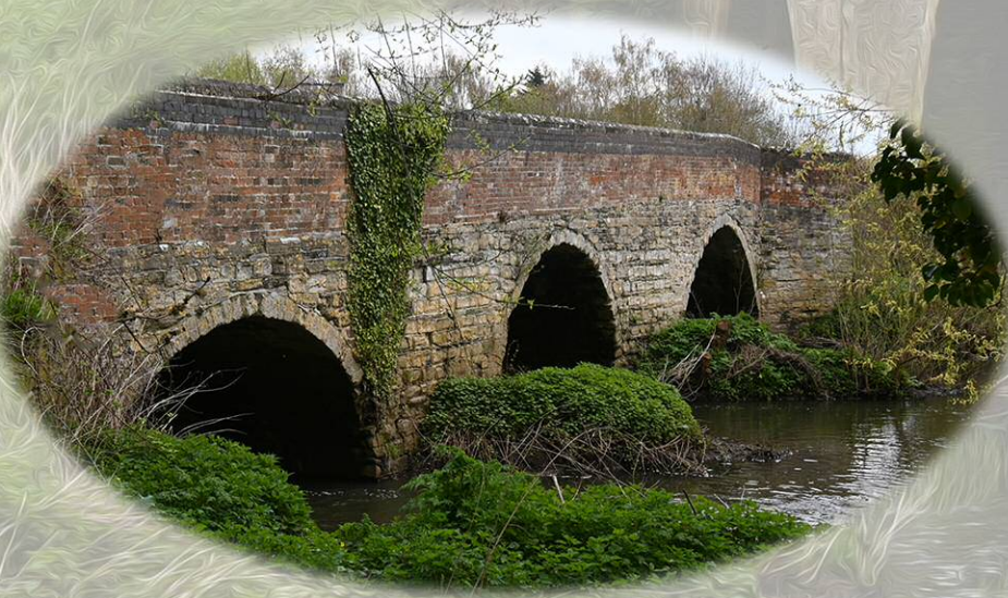
South side of the bridge in 2023.
